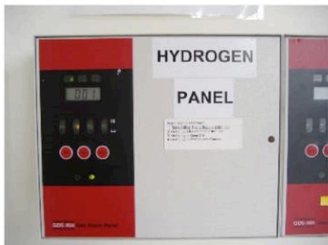
Figure 1. Hydrogen Detection Control Panel
